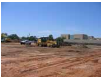
Construction is underway on the new SOP in Abilene.
