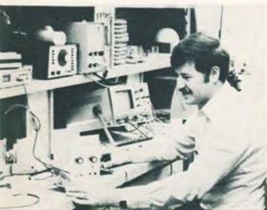
Grad Student Leon Shturman builds and tests a neurostimulator designed during an academic course.
