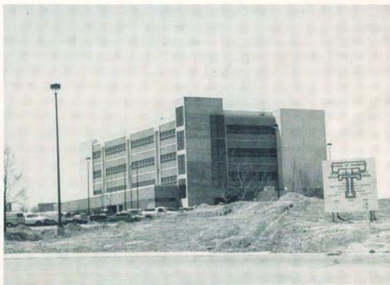
TTUHSC School of Pharmacy under construction in Amarillo
