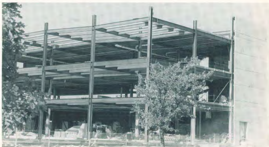
Side view of library construction
