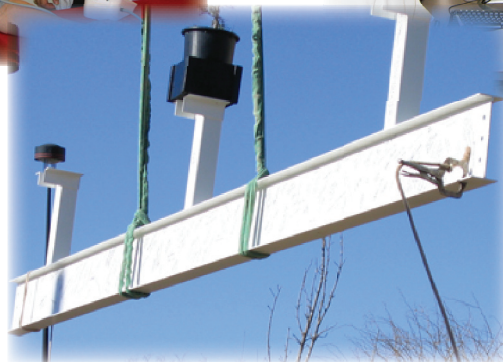
The final beam for the Amarillo Research Building is hoisted into place at the Topping Out Ceremony.
