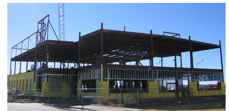
Construction is underway at the TTUHSC Research Building in Amarillo.
